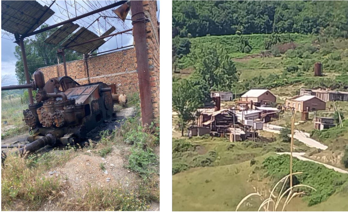
Fig. 2. View from the petroleum refinery of the case study
